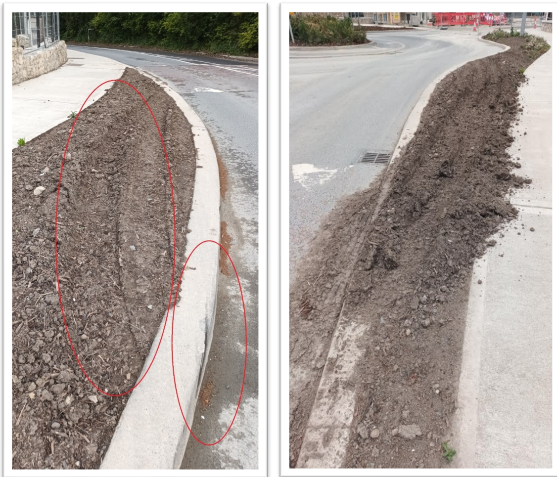
Fig. 6 Kerbing and overrunning on footpath at Brennanstown Wood (regular occurrence).
